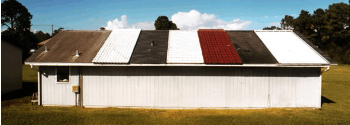
Figure 2. FSEC Flexible Roof Facility showing roof/attic test cells under test. The 2 test cells with the dark composition shingle roofs are the subject of this report.
